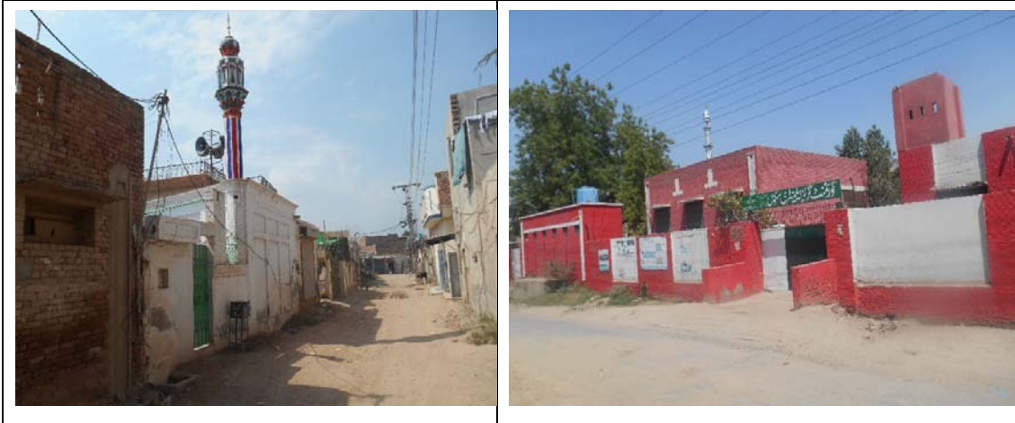
Pictorial view of Force main Line from New Disposal Station Site to Sewerage Drain, Kamalia
