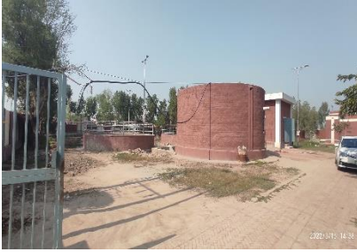
A view of collecting tank at nawaz sharif disposal station
