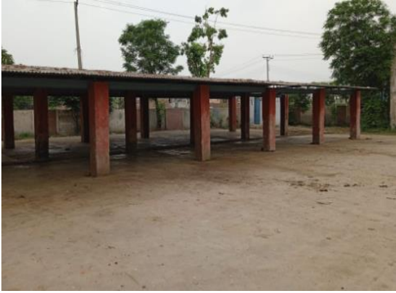
Figure 23: Front view of Slaughterhouse
