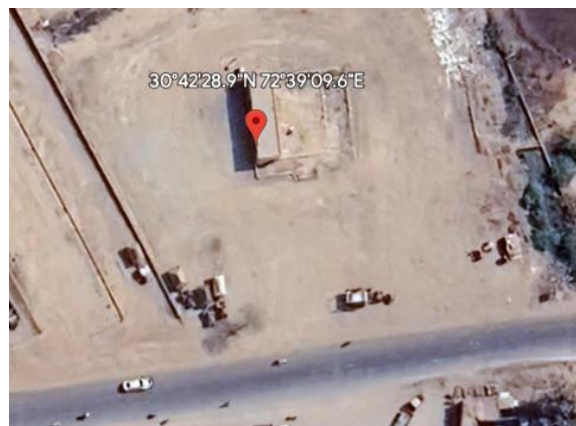
Figure 22: Aerial view of the Bus Stand
