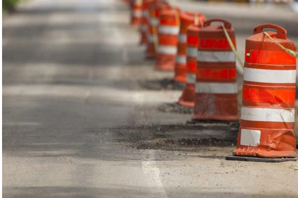
Figure 14: Traffic Diversion while road Repair
