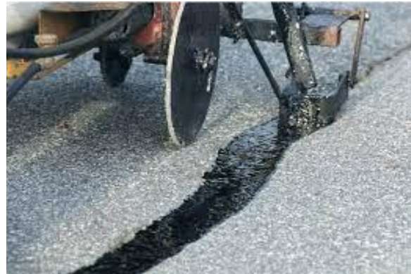
Figure 9: Repair of Cracks using Saw and Seal Method
