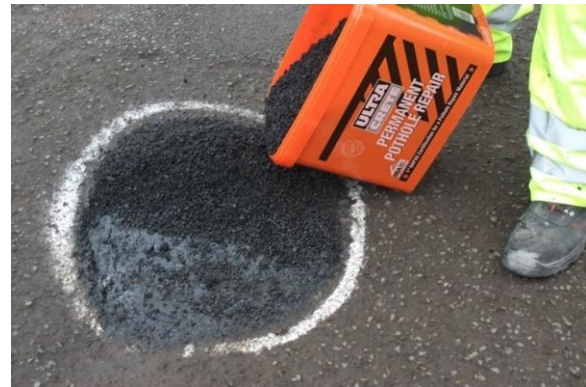
Figure 7: Repair of pothole
