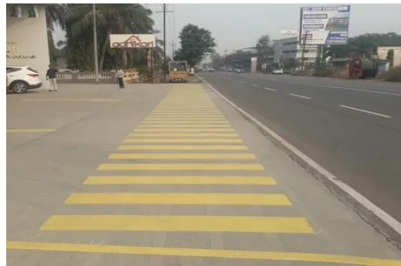
Figure 13: Proper Marked Road
