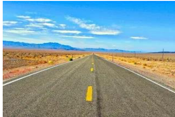
Figure 3: Water-Bound Macadam Road
