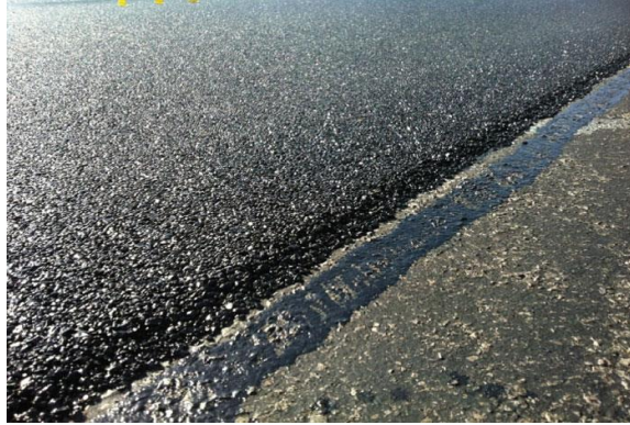
Figure 10: Thin Overlay on existing Road
