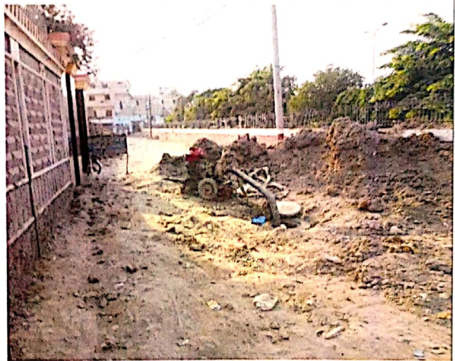
Sewerage Rehabilitation near Fazil Deewan
