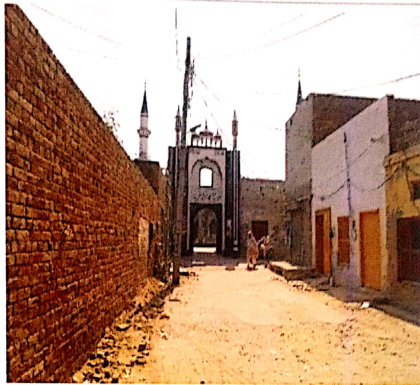
Poor Road Condition near Jamia Masjid Ghosia
