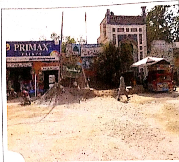
Poor TST Road at Eid Gah Chowk
