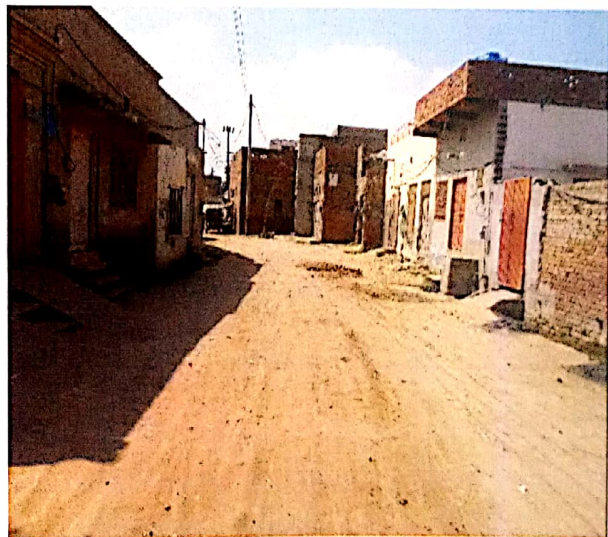
Worn TST Road near Mohallah Fazil Deewan
